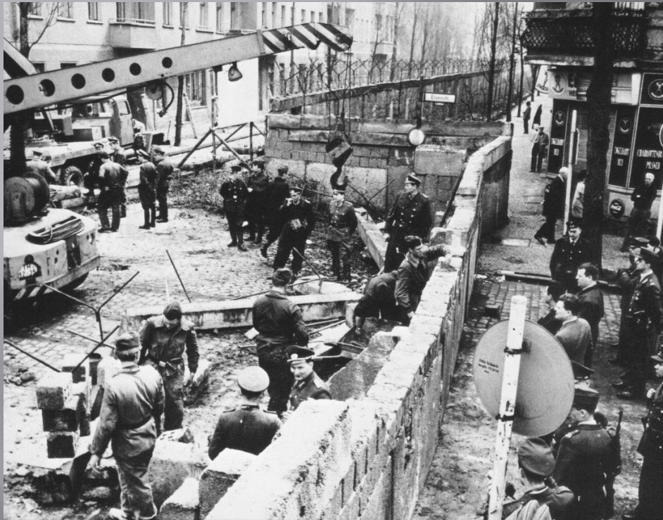
Building the Berlin Wall, Aug. 1961
